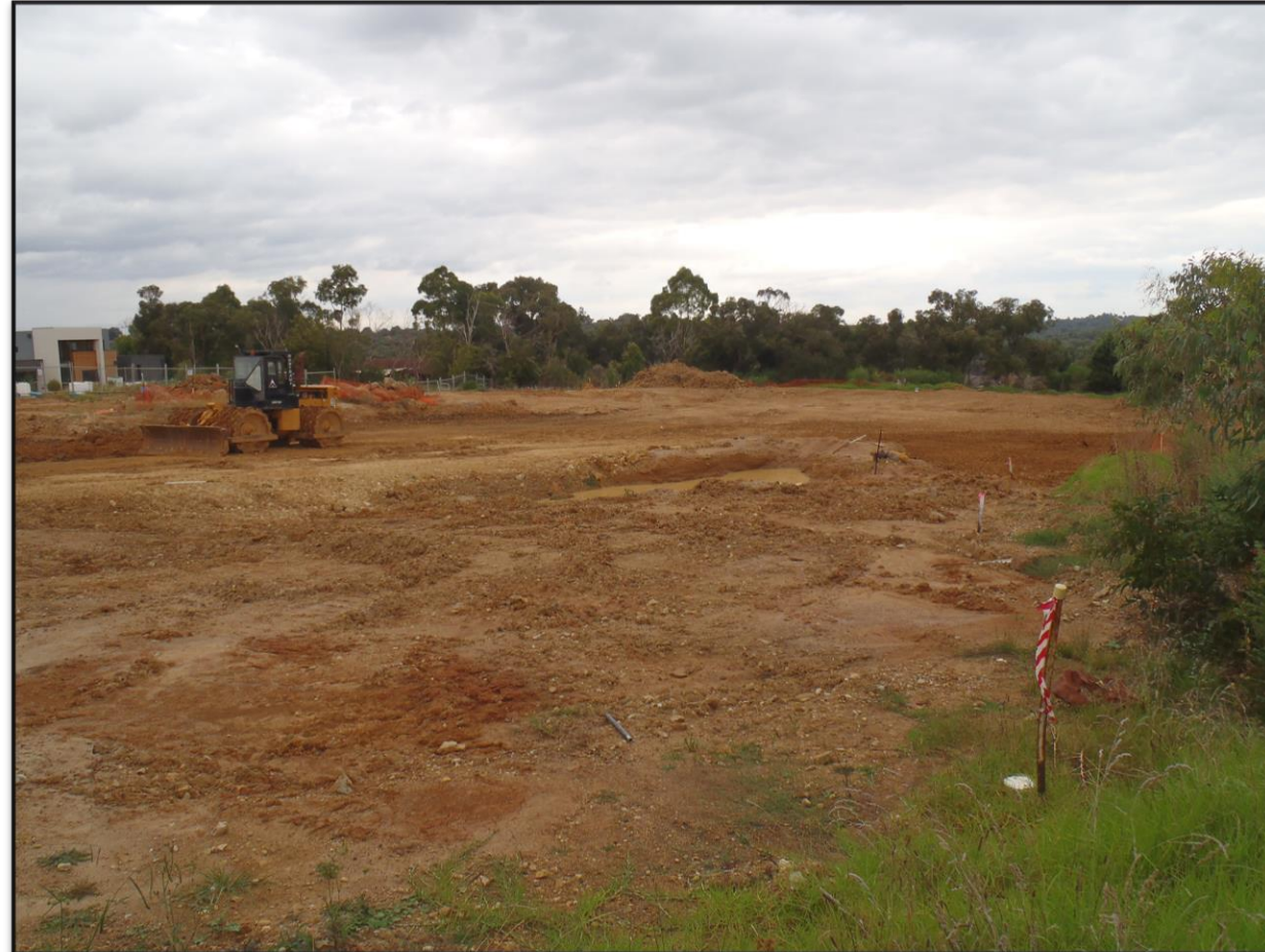
Backfilled Excavation Following Remediation
